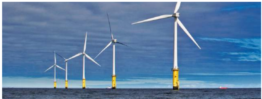
A photo of North Hoyle Offshore Wind Farm where the turbine height measurement from sea level to blade tip is 107 metres. The height to the tip of the blades at Triton Knoll Offshore Wind Farm would be a maximum of 220 metres from sea level.
