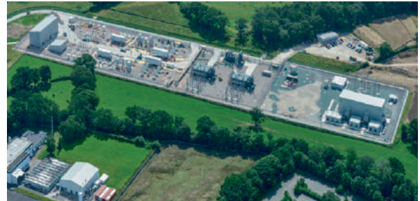
Gwynt y Môr substation
