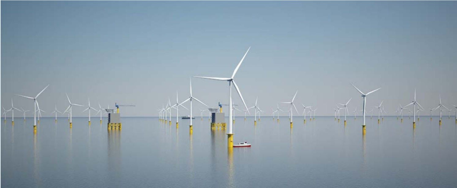
A computer generated image showing what part of the Triton Knoll Offshore Wind Farm could look like based on 288 125 metre tall turbines.
