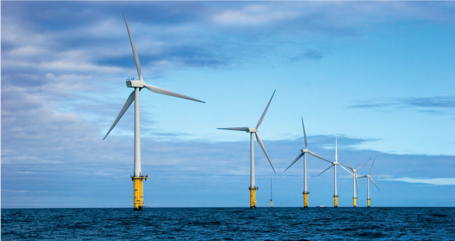
RWE npower renewables' North Hoyle Offshore Wind Farm. This photo is not intended to represent the appearance, size or scale of the proposed Triton Knoll Offshore Wind Farm.
