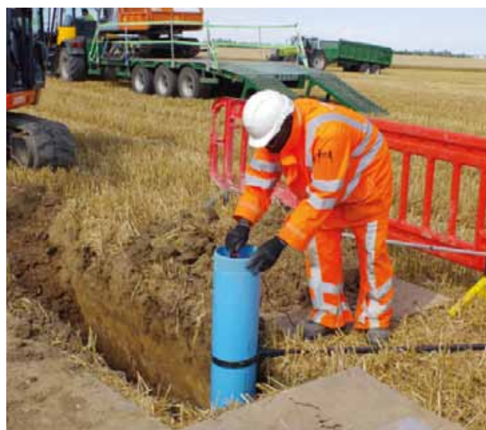
Photo: A trial trench from the recent Site Investigation campaign.
