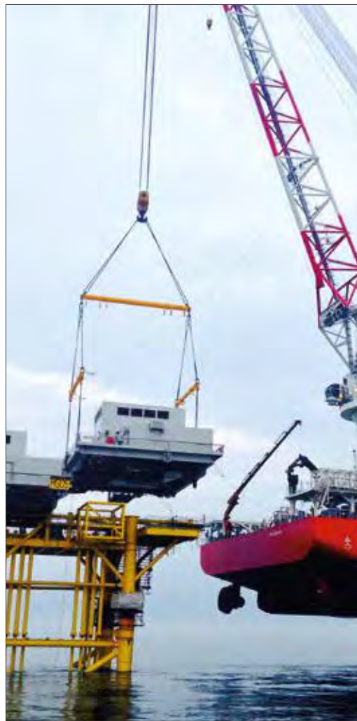
Construction of a substation at the Humber Gateway project. The jack-up barge's crane lifts the substation components into place.
