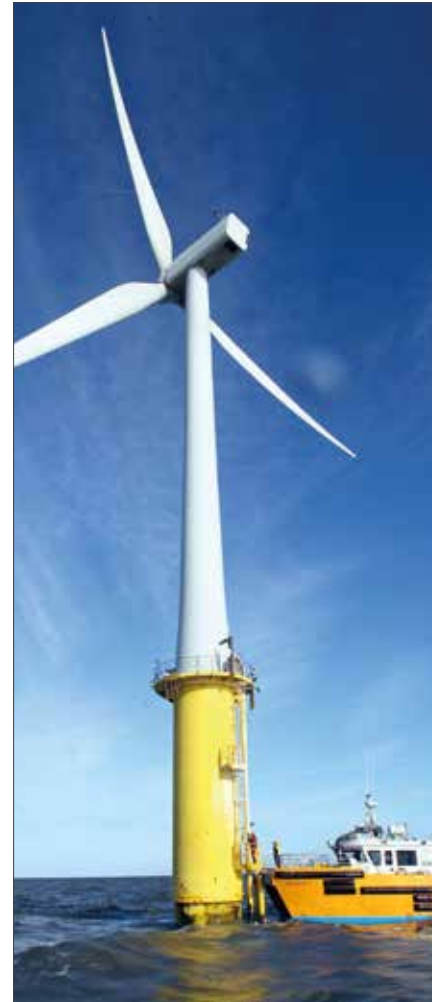
A turbine on a monopile foundation at North Hoyle—the first full-scale offshore power plant in the UK. The crew transfer vessel is seen docking at the transition piece access ladder.
